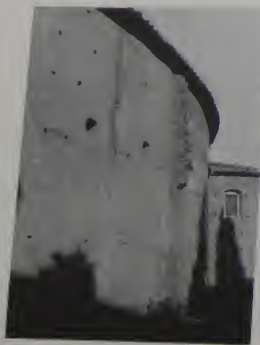
Fig. 178. S. Stepha. Rotunda. Arrangement of brick (upper) and T-pier masonry (lower).
